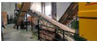
Reference: MZA-005 CONVEYOR BELT Year: 2018 Brand: TREICO
